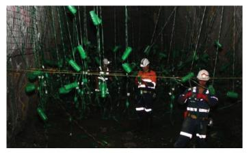
Loading electronic detonators in production charging.
